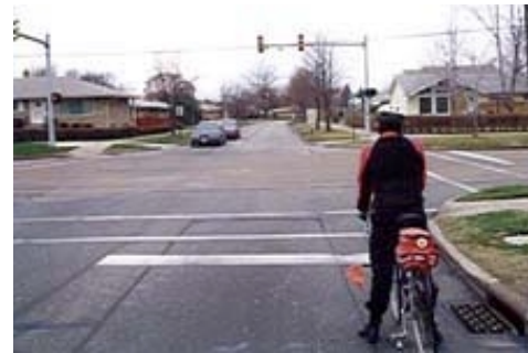
Simple Loop Detector: Detector wires are under the cyclist's left foot and also near left side of lane. (He should be further left.)
