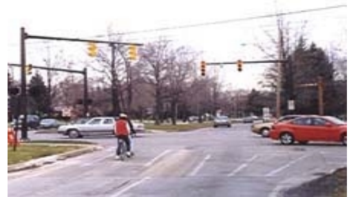
Double Loop Detector: The bike is over the "hot spot" in the center of the left turn lane. (The cut marks in the right lane are easier to see.)
